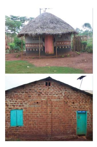
Figure 1. Typical hut built with adobe construction and. typical mud-brick construction
